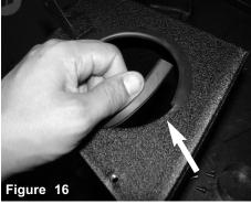
Install the vinyl trim to the hole in the heat shield ...
